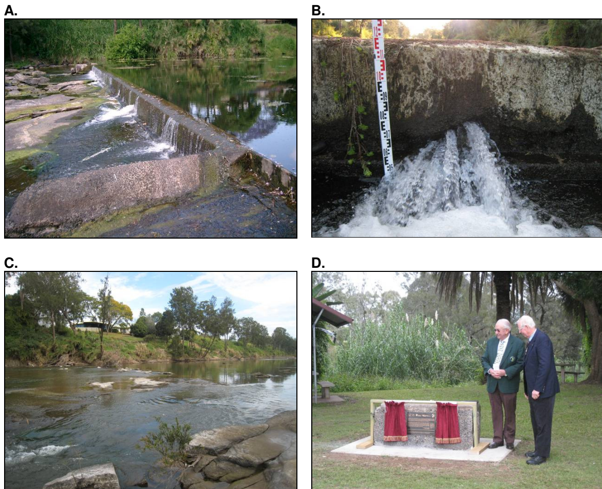
Figure 1: A. Manyweathers Weir restricted fish passage to over 1000 km of waterway in the Richmond catchment. B. State Water Corporation considered the weir redundant, with multiple breaches limiting the weir's capability to pool water during drought conditions. C. The weir was removed in its entirety in 2009, with a section of the weir maintained to honour Richmond Manyweather (D).
