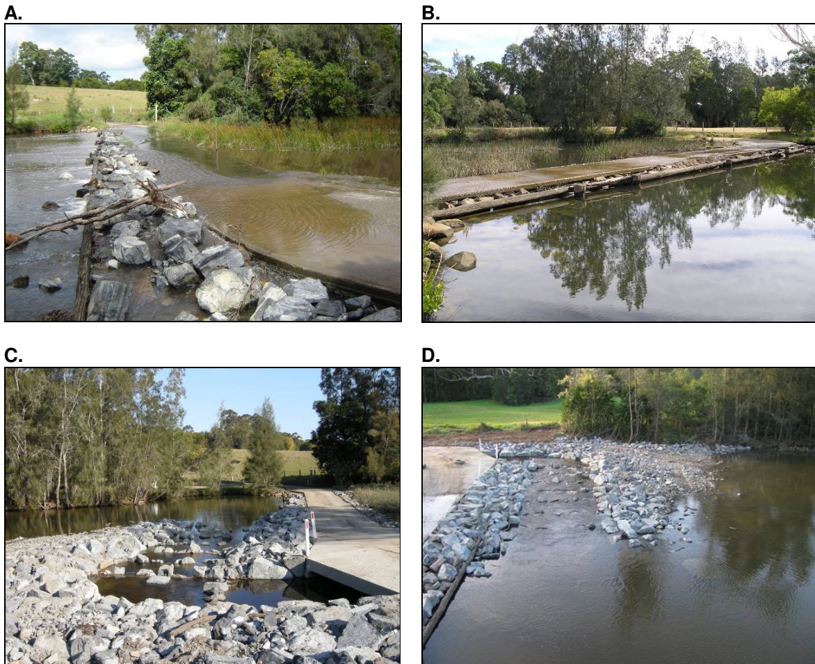
Figure 3: A & B. Locketts Crossing restricted fish passage to over 60 km of upstream habitat due to excessive headloss. C & D. A partial-width rock-ramp fishway was installed on the downstream side of the crossing that led to a single box culvert.
