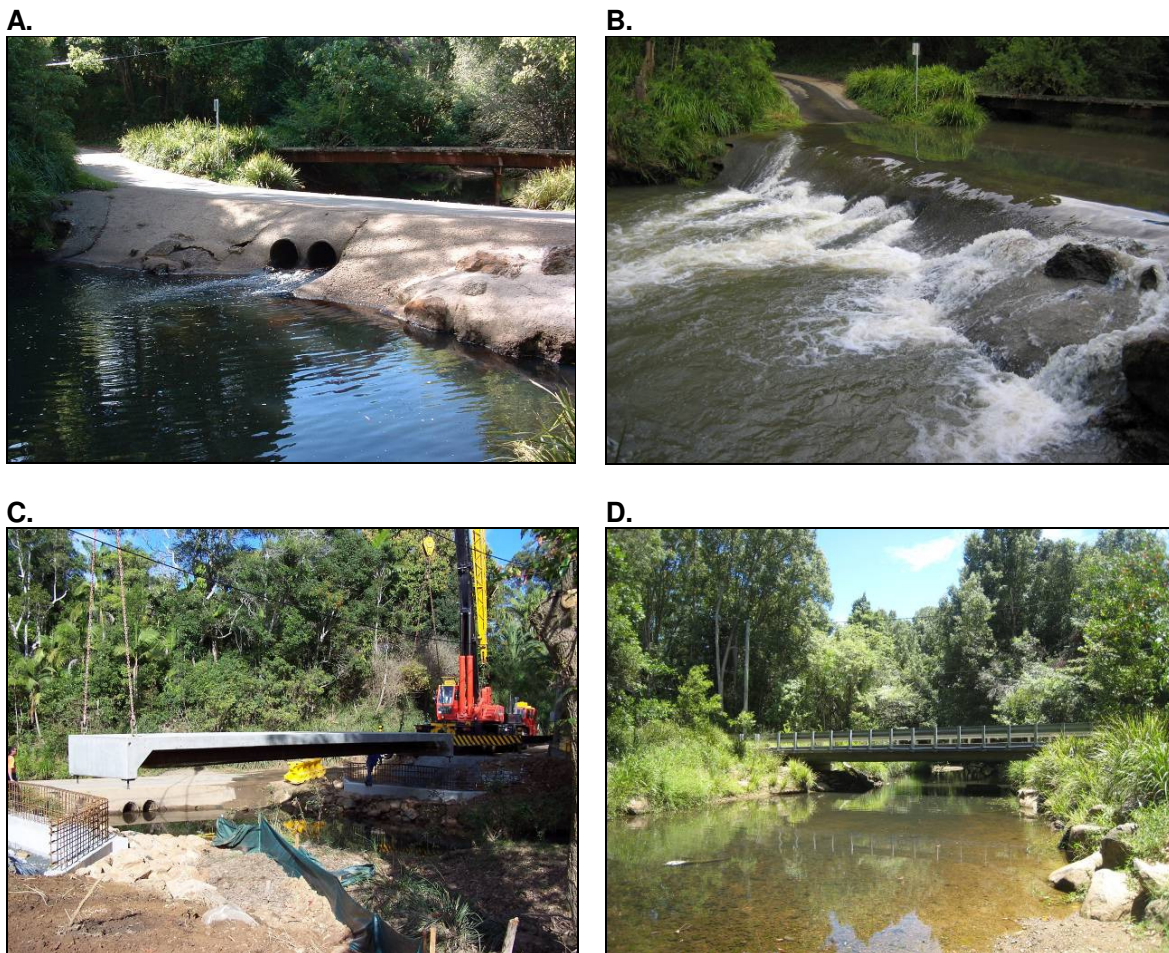
Figure 2: Coral Avenue causeway restricted fish passage during base flows due to high velocities through the two pipe culverts (A), and during elevated flows due to excessive head differential (B). C) Prefabricated Doolan Deck bridges were craned into place, thereby reducing onsite construction costs by up to 50 %. D) Coral Avenue bridge provides improved fish access to over 25 km of upstream habitat.
